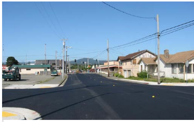
Construction on Fifth Street included overlays and pedestrian improvements.
