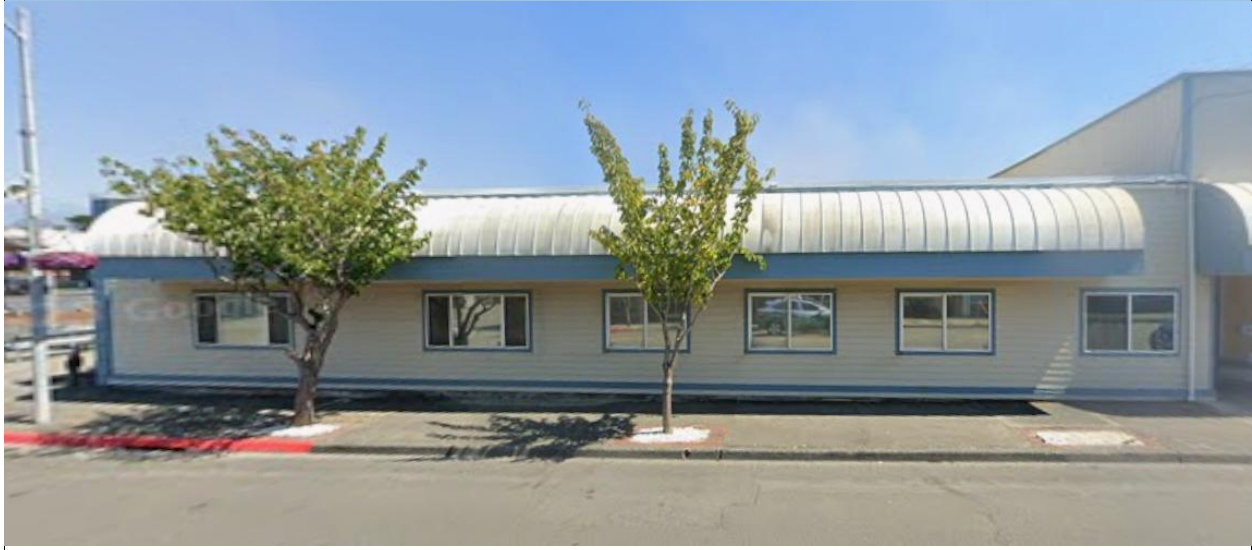
Source: Google Street View (July 2025)
