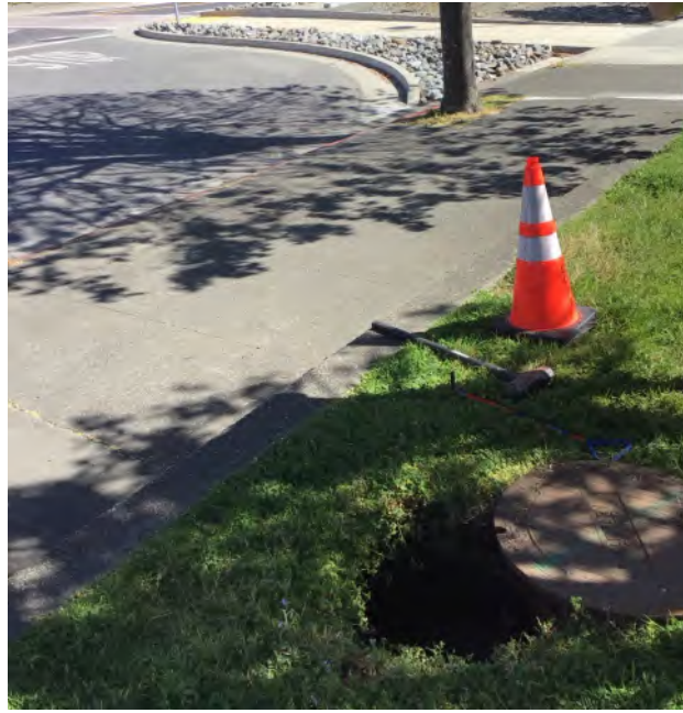
Figure 9.20 Manhole investigated during data collection near Front St.
