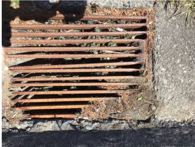
Figure 9.22 Grate inlet found in field data collection.
