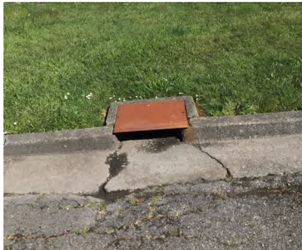
Figure 9.21 Curb inlet found in field data collection.
